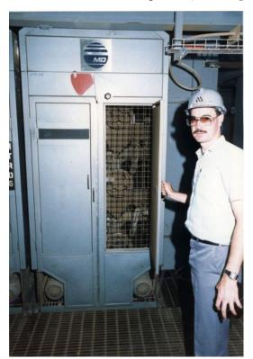
Figure B.5.: Enclosure around a HTR Separator, showing inspection door
