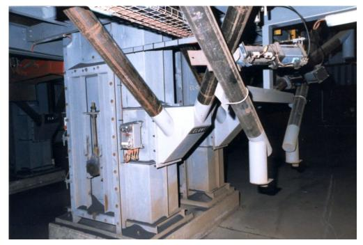
Figure B.9.: Enclosures around bucket elevator feed points
