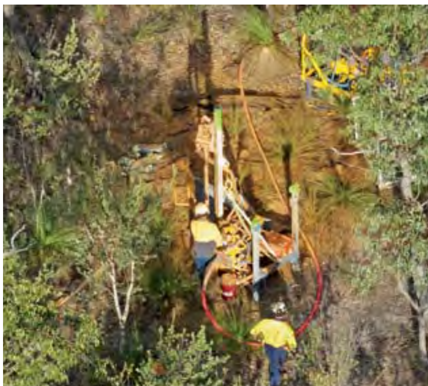
Drilling shot holes to provide optimal recording parameters for the Wannamal 3D Seismic Survey over the Gingin Gasfield area and Wannamal Prospect (Photo courtesy of Empire Oil and Gas)
