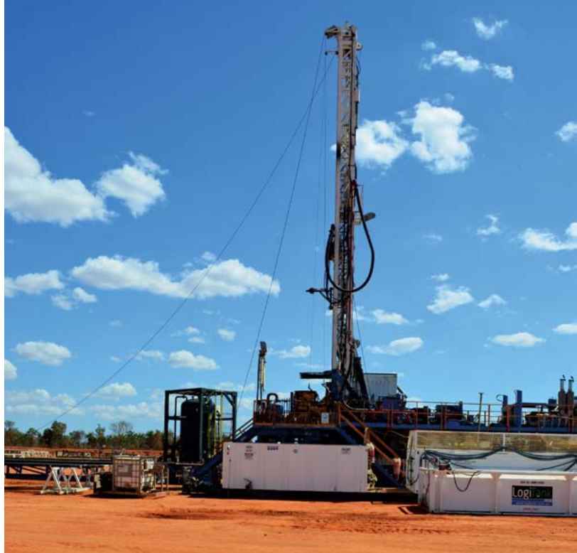
Altas Rig 2 at Prasin 1
