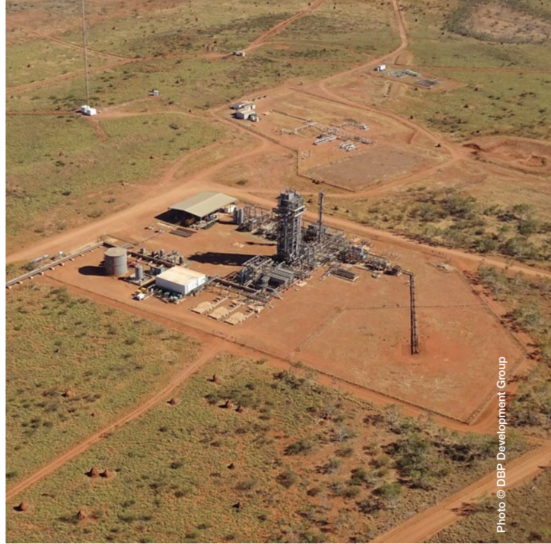
An aerial view of the new Tubridgi gas storage facility
