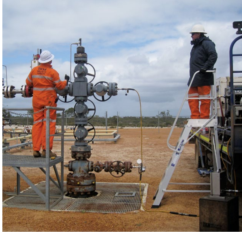
Conducting a well integrity test
