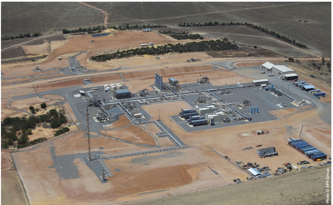
Aerial view of the Mondarra gas storage facility
