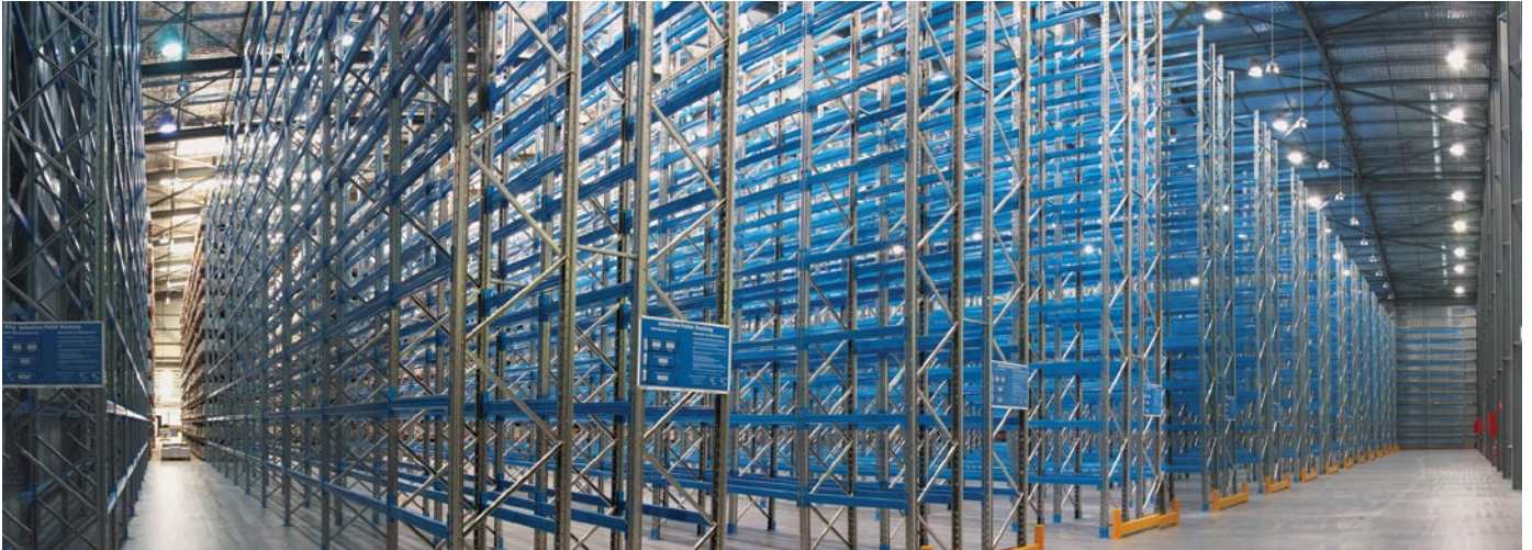
Pallet racking at the Perth Core Library
