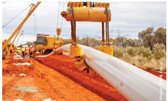
Laying of pipe in the trench
