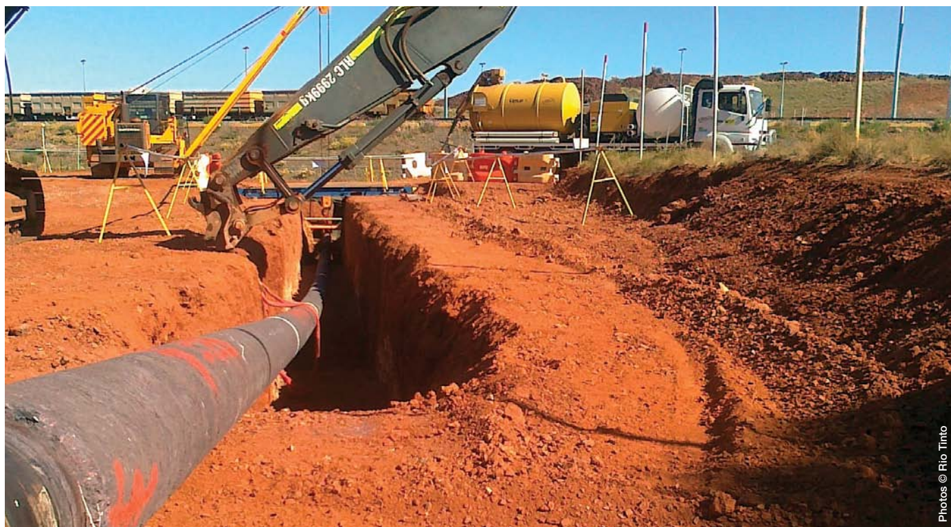
False trench for the 188 m rail crossing
