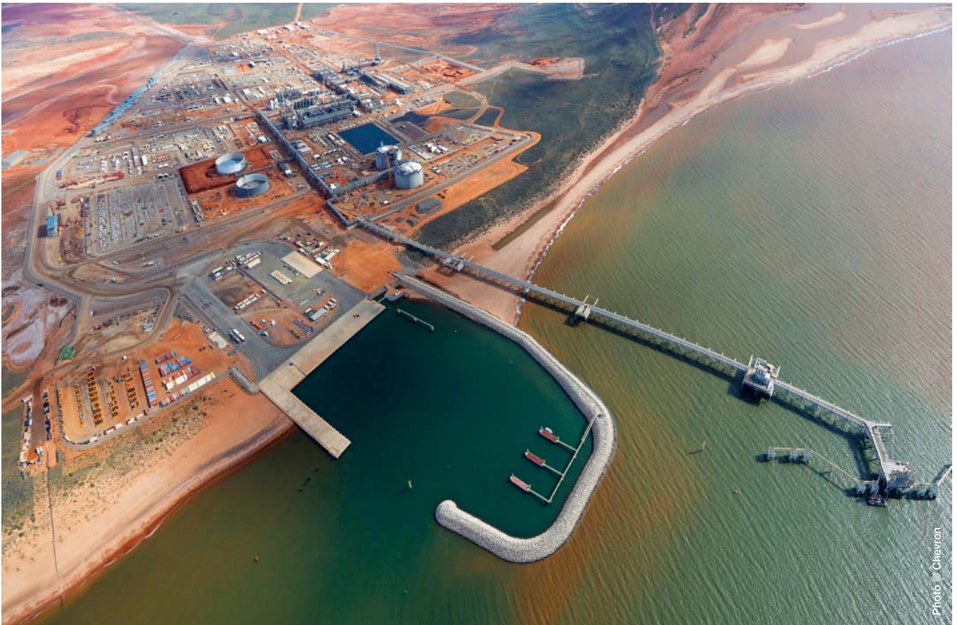
Aerial view of the Wheatstone Project LNG Plant at Ashburton North
