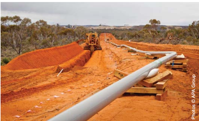
Trench construction and welded pipe
