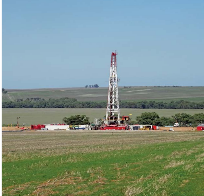
Onshore drilling in Western Australia
