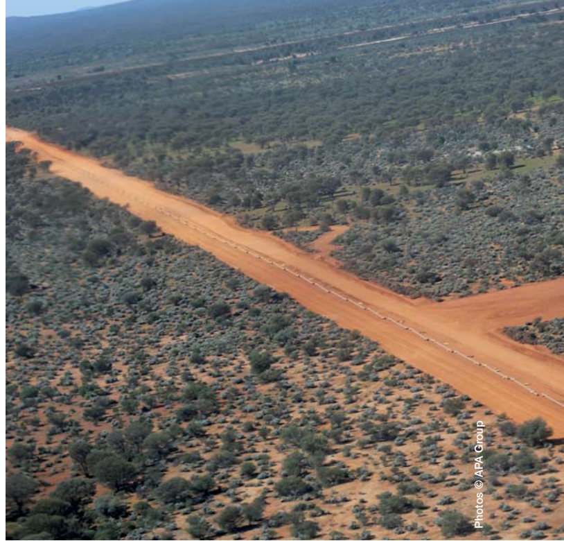
Pipe laying for the Eastern Goldfields Pipeline
