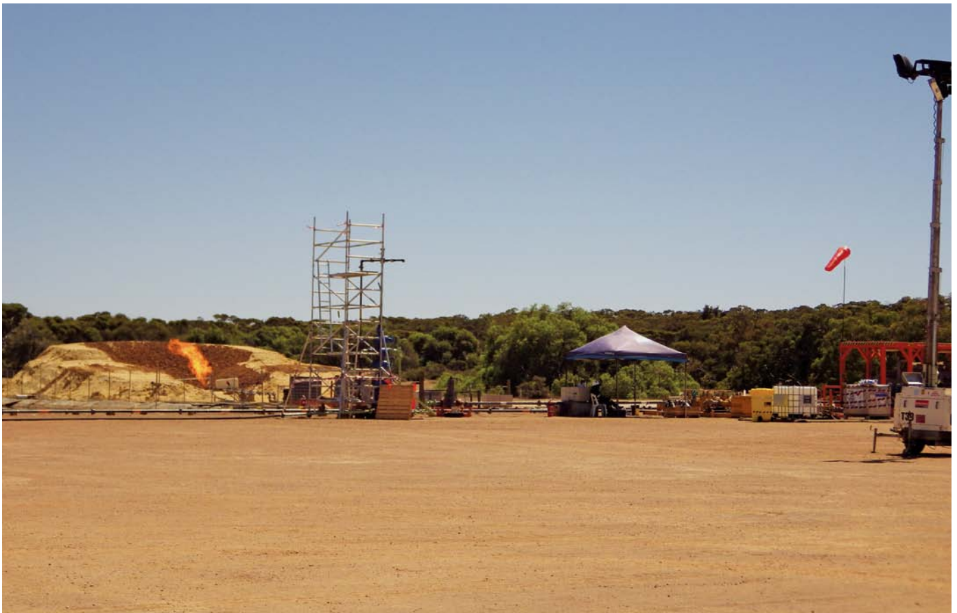
Well test at Warro 5
