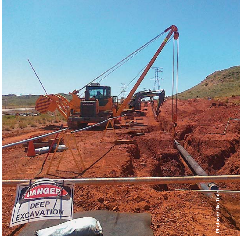
Lowering in the pipeline
