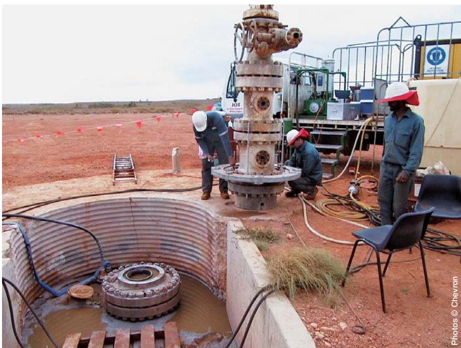
Decommissioning a well – removing the Christmas tree
