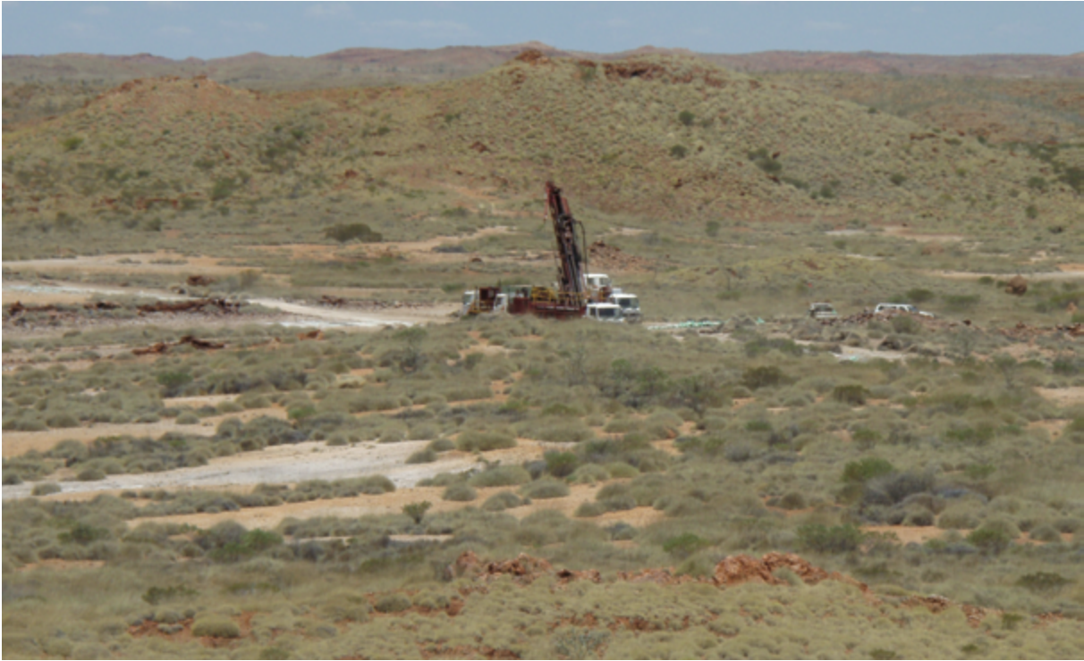
Figure 17.1 When setting up an area for hot work, consider where sparks might be carried by the wind. Choose a location that minimises the risk of fire and can be seen by other crew members. Before starting any work that may generate sparks, ensure you have adequate fire-fighting resources for emergency use
