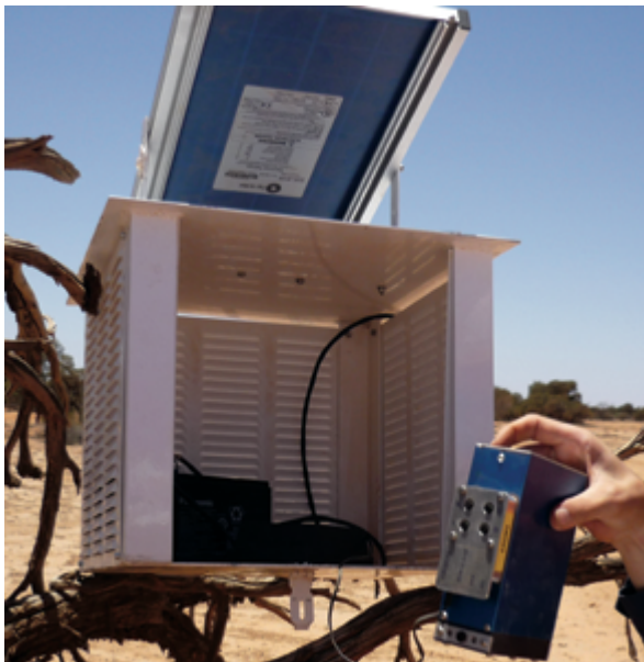
Figure 16.2 Example of radiation monitoring station
