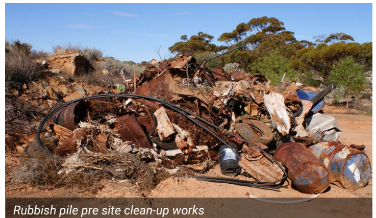
Plant area following infrastructure removal
