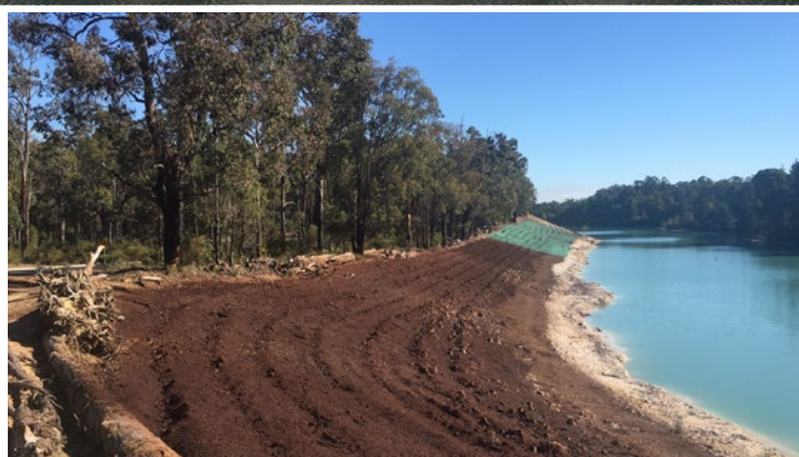
The application of growth medium on the slope.
