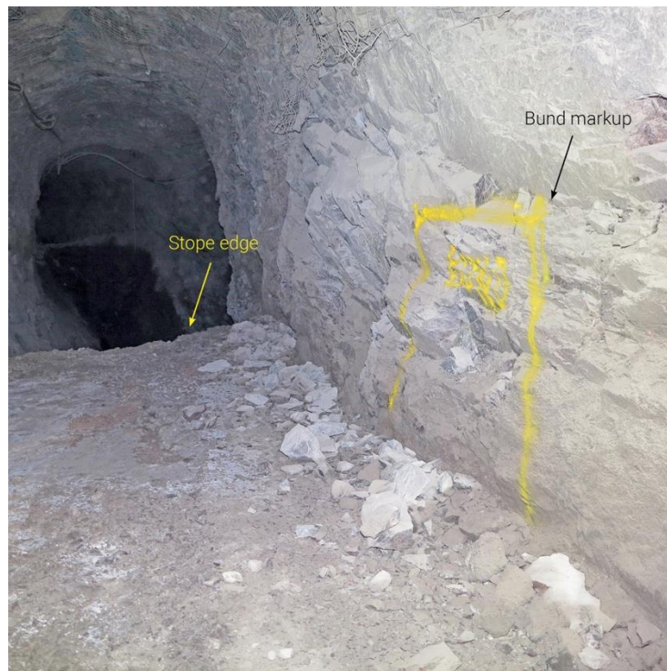
Photograph of bund marking and stope edge
