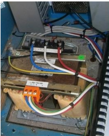
Left: Control transformer with exposed 1000V terminals. Centre: Tiny hole in glove. Right: Wrist of injured worker.
