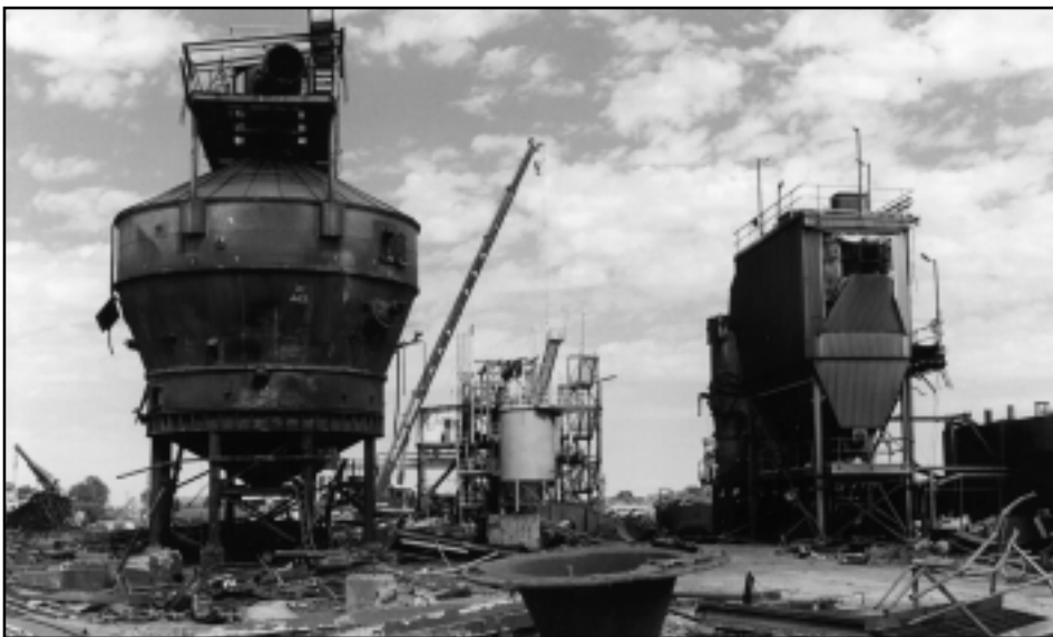
Demolition in progress.
